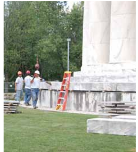
State capital appropriations financed restoration of the Harding Memorial, which was completed by September 2009. Workers are in the process of relaying the pavers on top of the base of the tomb to help eliminate staining on the base.
