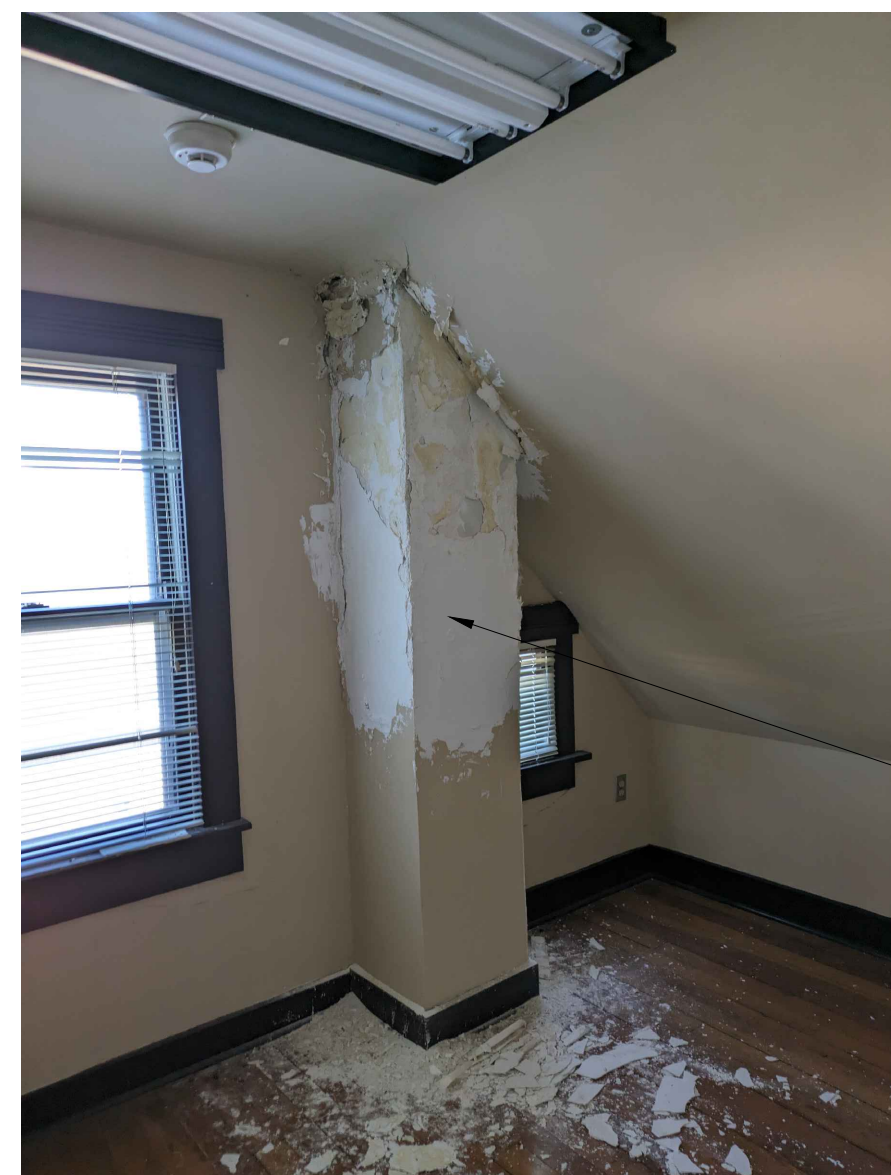
WEST WALL, WEST ROOM, 2ND FLOOR
