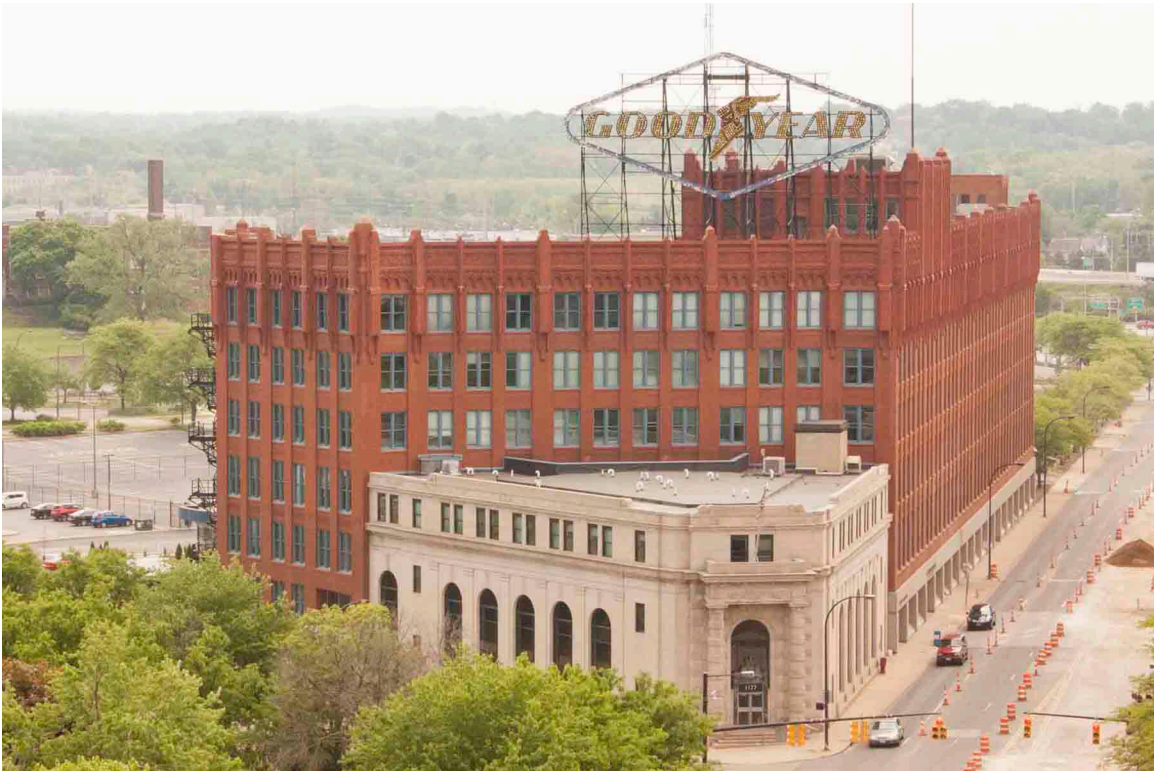
1. Front façade looking south east
