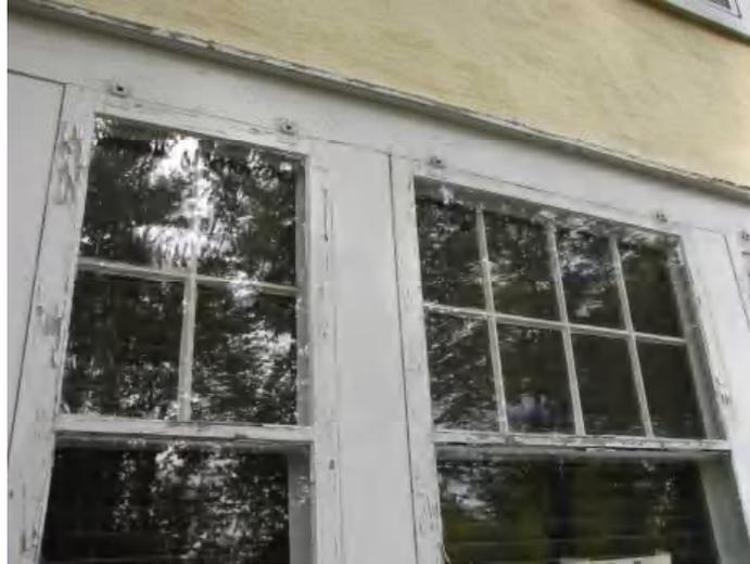
This Brookfield house has double-hung sash windows that combine a single-pane lower sash and multiple-pane upper sash. This was a common window type used when early 9<sup>th</sup> century homes were renovated in the early 20<sup>th</sup> century. Note also the traditional wood storm windows, hung from hooks just above the window, with a tight fit in the window opening to cut down on cold air infiltration.
