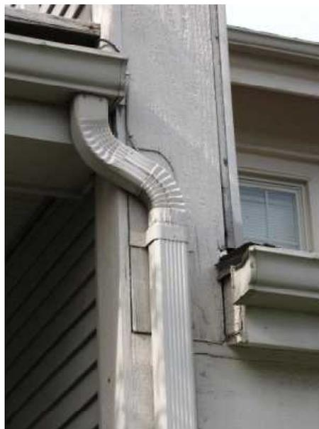
**Gutters and downspouts have the critical job of catching water from the roof and carrying it down to the ground. Curved connectors like this one often have to be installed on a building, but they can easily plug up with debris and must be watched carefully and cleaned out right away when they stop working.**
