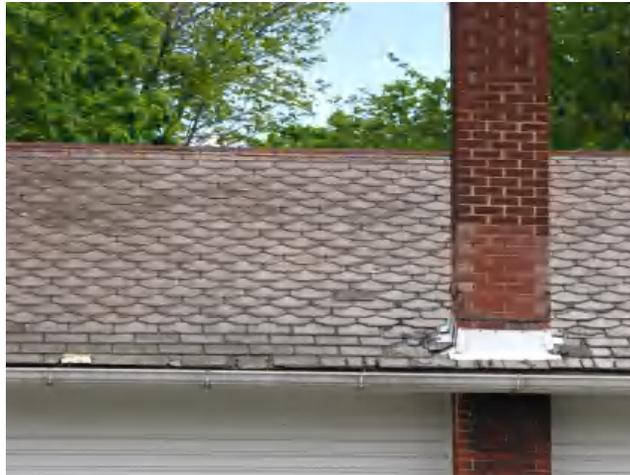
The roof is the first line of defense in the battle to keep water out of a building. This original slate roof has many years of service life left, but it must be cared for properly. The most important things to do are to replace or re-install any missing or dislodged slates; and to avoid walking directly on the roof surface while doing work.
