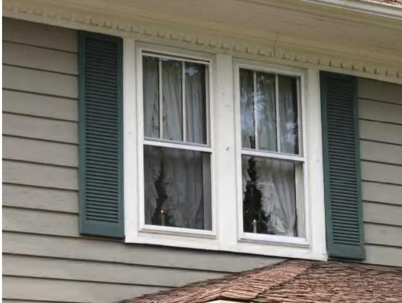
These windows are original to the early 20<sup>th</sup> century house where they are installed. They are "three-over-one" double hung sash windows. They have modern storm windows that have a minimal visual impact, with a dividing bar directly in front of the meeting rail of the window sash.
