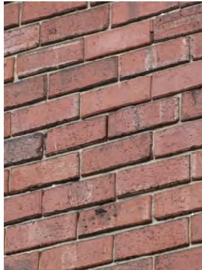
This Brookfield commercial building has a brick exterior with "raked" mortar joints. The mortar is recessed close to half an inch to accentuate the shape and pattern of the bricks. This was done on purpose as part of the overall design; any future re-pointing should keep the raked mortar joints. Raked joints accentuate the shows made by the bricks in a wall, giving the wall strong texture and a distinct look.
