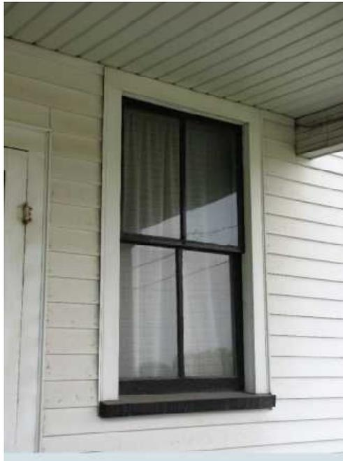
Brookfield is fortunate to have several buildings with original historic wood windows. This is an example of the classic "two-over-two double-hung sash." This means that the upper and lower sash have two glass panes each, and that both sash move independently up and down in slots. In such windows, the upper sash is always offset outside the path of the lower sash.
