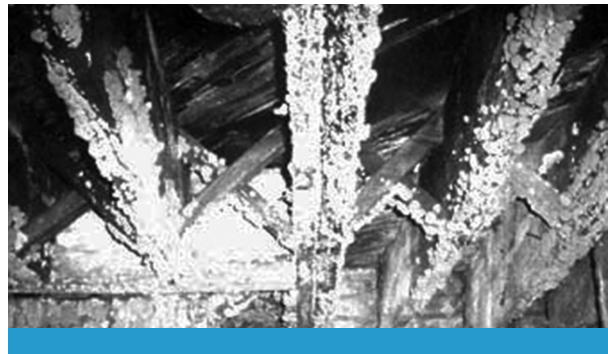
This is advanced wood rot. Note the fungi's fruiting reproductive bodies on the wood members.
