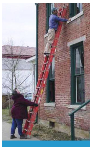
Careful use of an extension ladder
