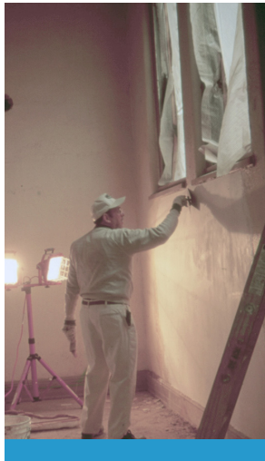
Plaster being repaired
