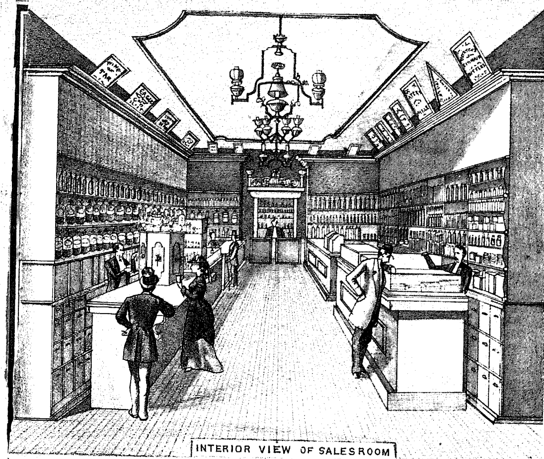
INTERIOR VIEW OF SALES ROOM W. F. HALE, CITY DRUGGIST AND APOTHECARY. CRATTON BLOCK, BROADWAY ST. JACKSON C.H. JACKSON CO. OHIO.
