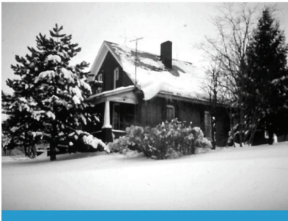
*Snow dams that formed on a poorly insulated roof*
