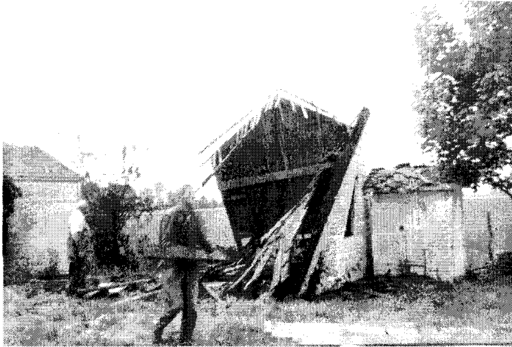
Figure 11. Orville Musselman dismantling of smokehouse, shed & privy, 1961.
