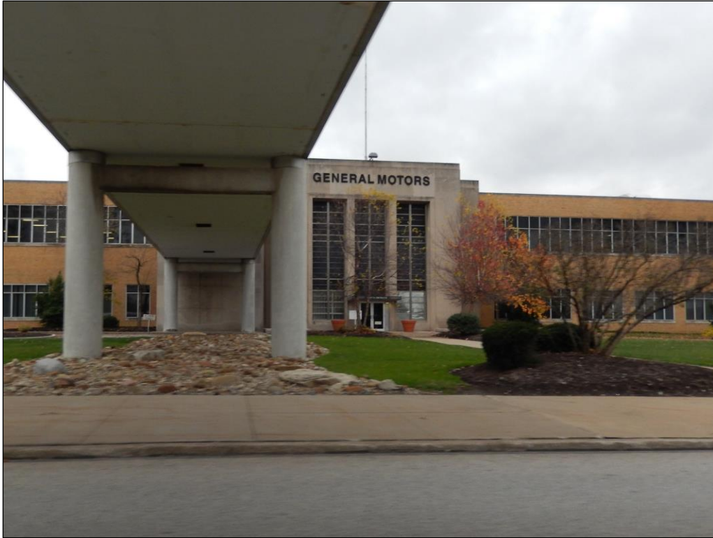
Plate 27. General Motors Fabrication Division (CUY 1141617), constructed in 1949, 5400 Chevrolet Blvd., Parma.
