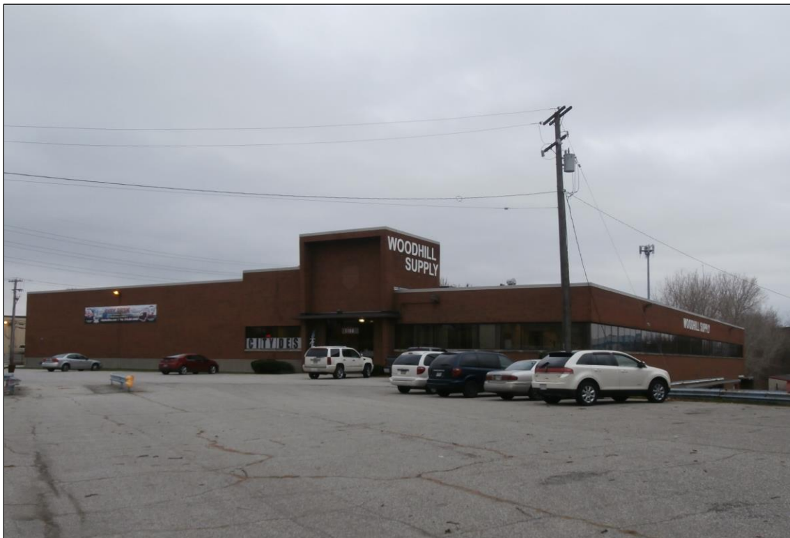
Plate 30. Former Graybar Electric Company (CUY 1110205), constructed in 1955, 1100 E. 55 th St., Cleveland.
