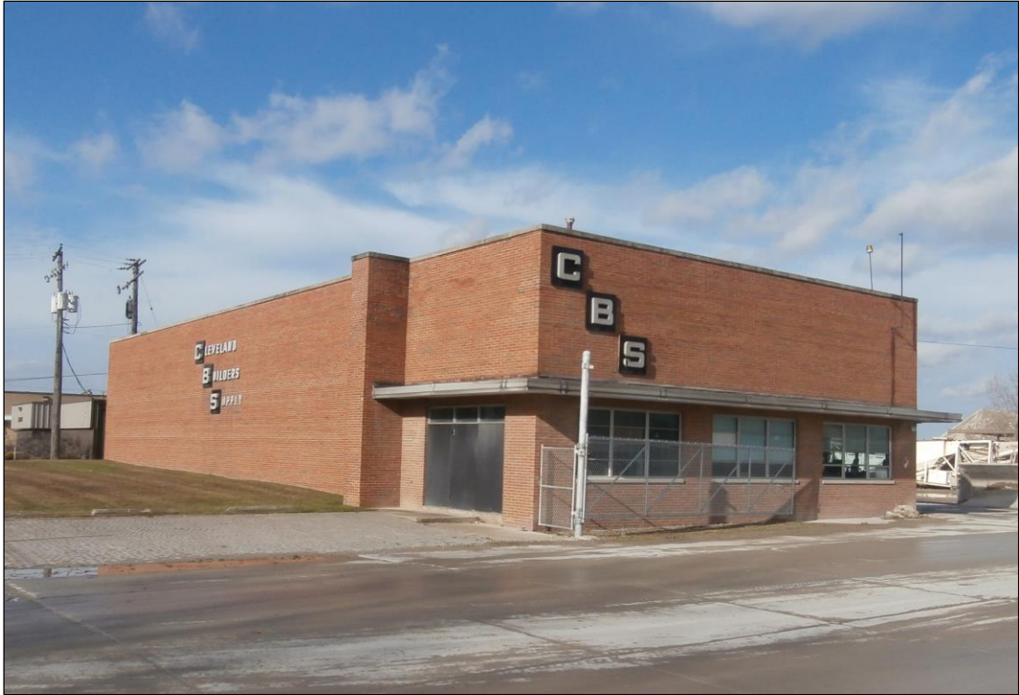
Plate 29. Cleveland Builders Supply (CUY 1105124), constructed in 1959, 26481 Cannon Rd., Bedford Heights.
