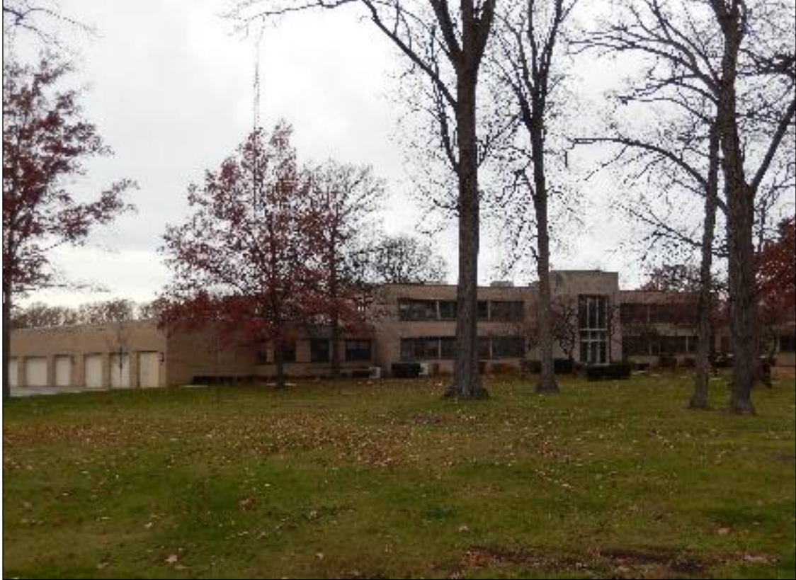
Plate 32. Rocky River Municipal Building (CUY 1158012), constructed in 1954, 21012 Hillard Blvd., Rocky River.
