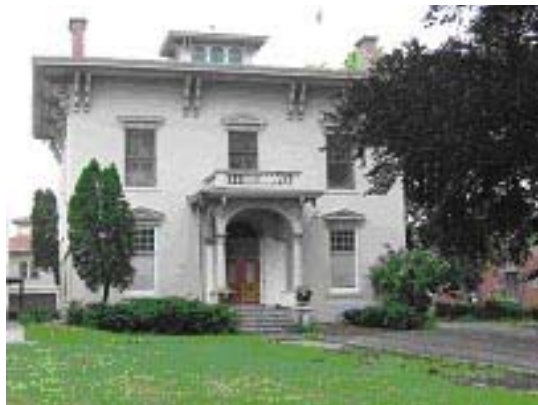
1857 Horace Starr House located in Washington Avenue National Register District. Currently being renovated for a History Center by the Lorain County Historical Society.
