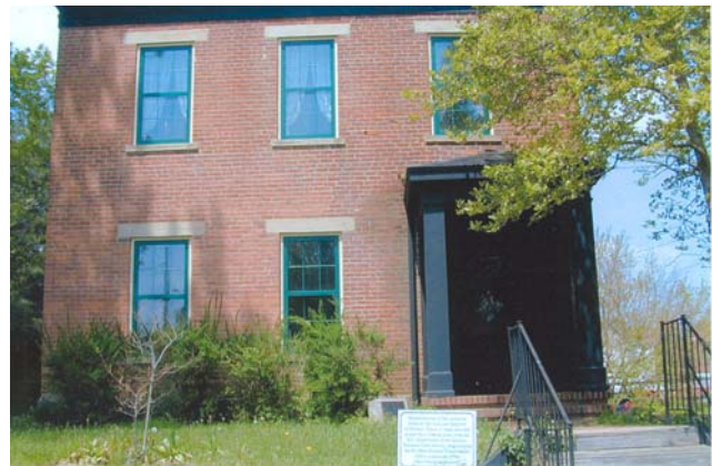
Ross-Gowdy House, window rehabilitation project, New Richmond.
