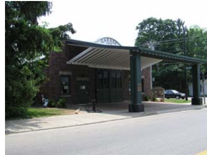
550 South Main Street, former 1919 Ford Motor service garage; currently The Garage youth center, an excellent example of adaptive use.
