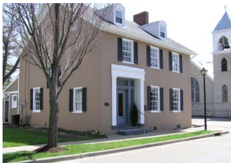
South Main Street streetscape
