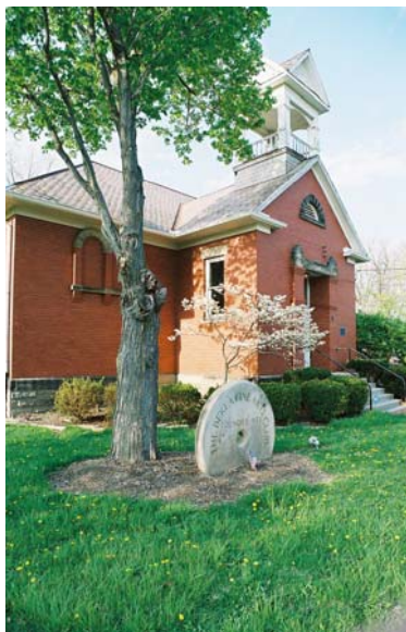
The restoration of Berea's Little Red School House for use by the Berea Center for Fine Arts, is being funded in part with a CLG grant.
