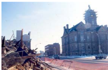
Demolition of Hancock County Jail and Sheriff's Residence.
