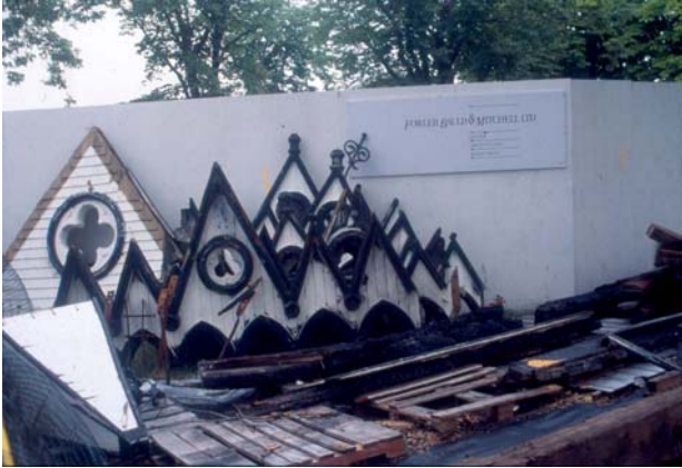
WOODEN ARCHITECTURAL ELEMENTS FROM A CHURCH HEAVILY DAMAGED FROM A FIRE WERE RECOVERED AND WERE INCORPORATED INTO THE RECONSTRUCTED BUILDING.
