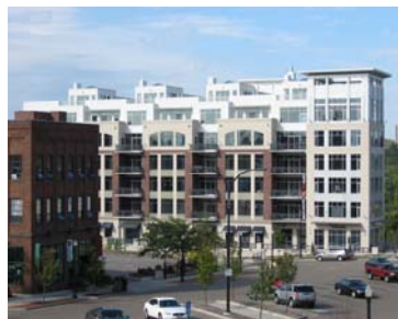
The new Northside Lofts Condominium project is fueling a resurgence in downtown Akron.
