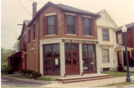
The restoration of the Wright Brothers Bicycle Shop in the Dayton Aviation History National Historical Park occurred after an historic photograph of the building was located.
