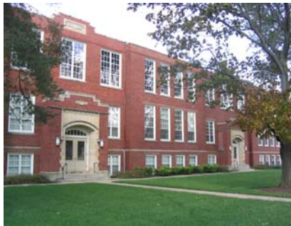
The former middle school now houses city offices.
