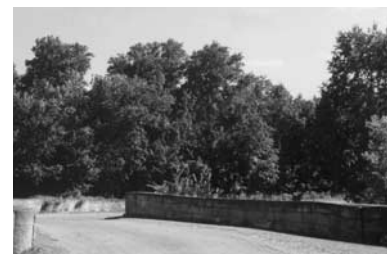
Salt Fork Creek S-Bridge
