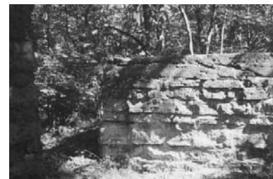
Miami-Erie Canal bridge footings at Tadmor, Montgomery County
