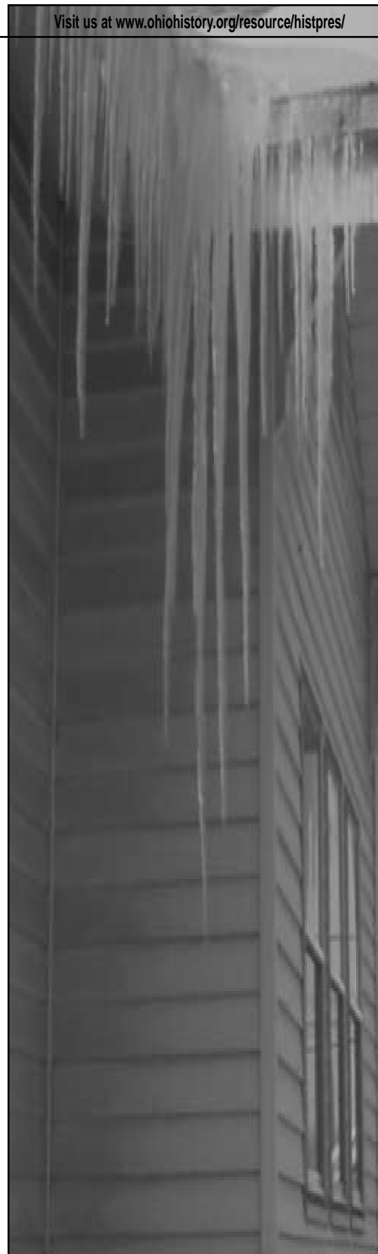
Dangerous icicles that have formed along unheated eaves.
