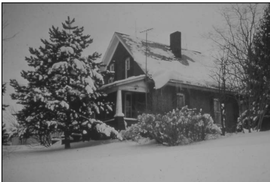
Snow dams that formed on a poorly insulated roof.
